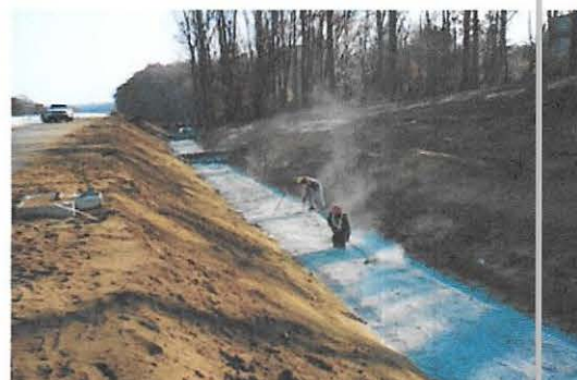
A new "water quality swale" along the NJ Parkway
