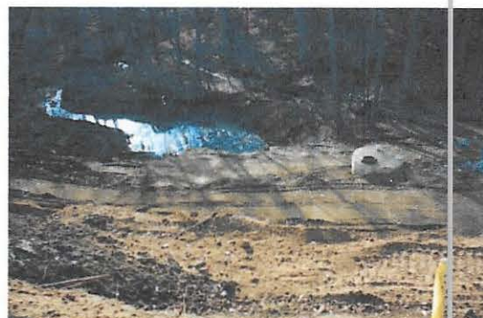
At the end of the swale, cleaner "filtered" water discharges into a stream
